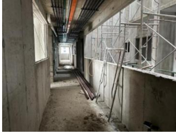
Figure 9. D'Quince Residence site location and condition
