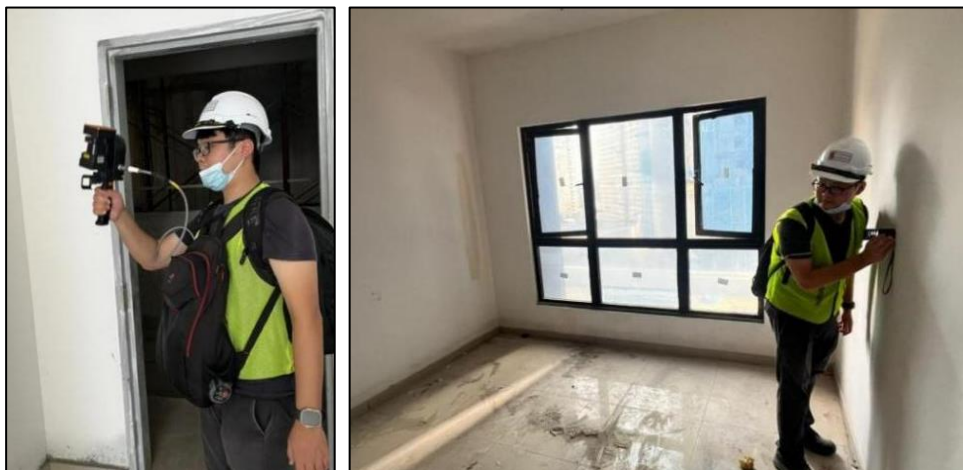
Figure 10. Data collection using HLS (Left) & As-built using distometer (Right)
