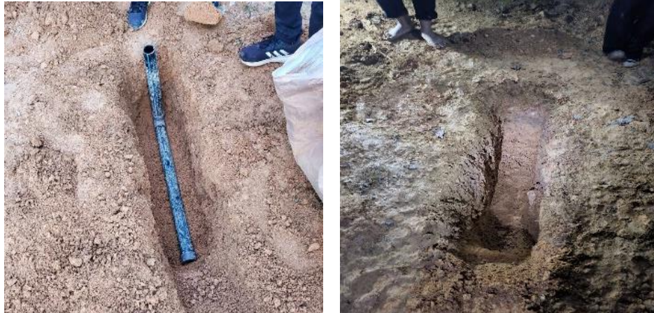
Figure 3. Pipe leakage test bed.
