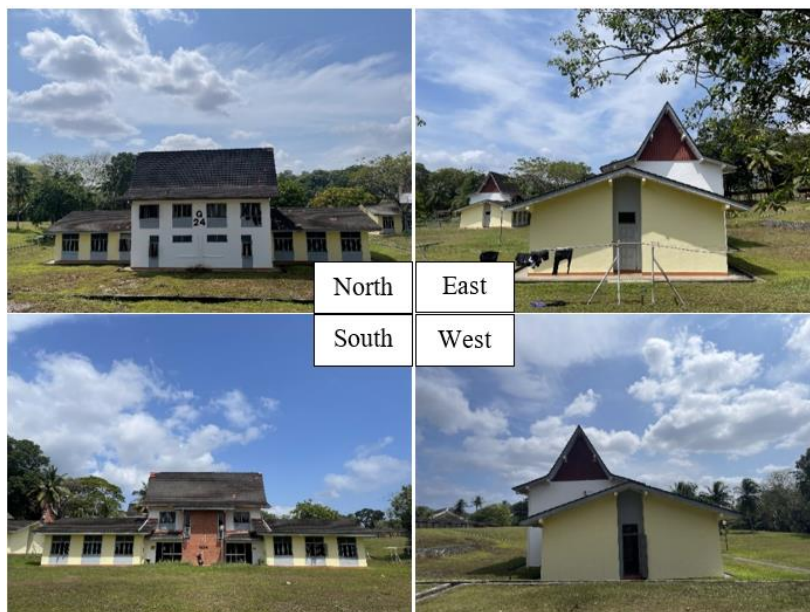
Figure 4. Close up of each site of building G24
