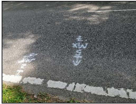
Figure 8. Depth was sprayed after detection by the locator
