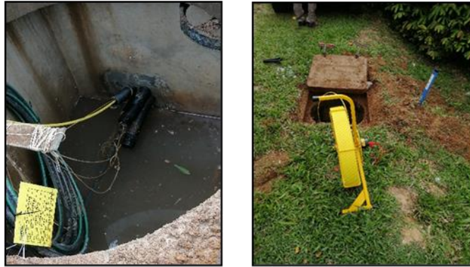
Figure 6. Duct road inserted into the jacket of fibre cable
