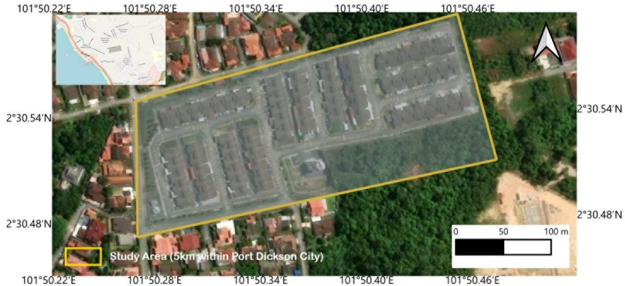
Figure 2. Construction site used as study area
