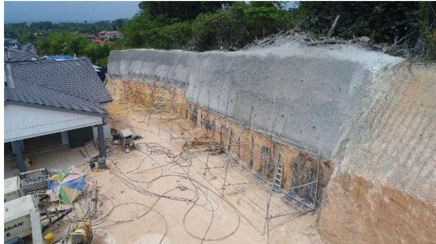
Figure 7. Gunite Application for Slope Stabilisation at Area 2
